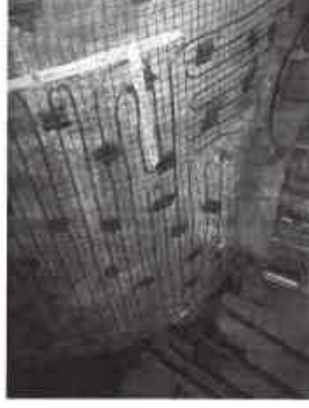
Electric heating coils to keep HP/ IP Turbine casing and shaft in warm start conditions
